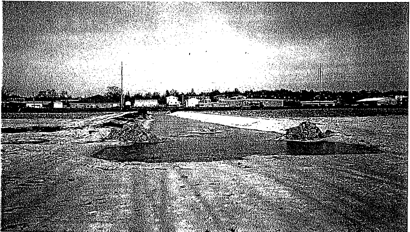
Above: Fill piles and weedy vegetation near Camp Cardinal Road at south end of JLS Property.
